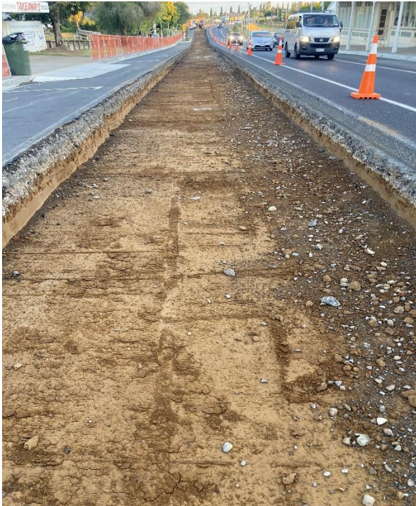
SH3 Ōhaupō during road rebuild
