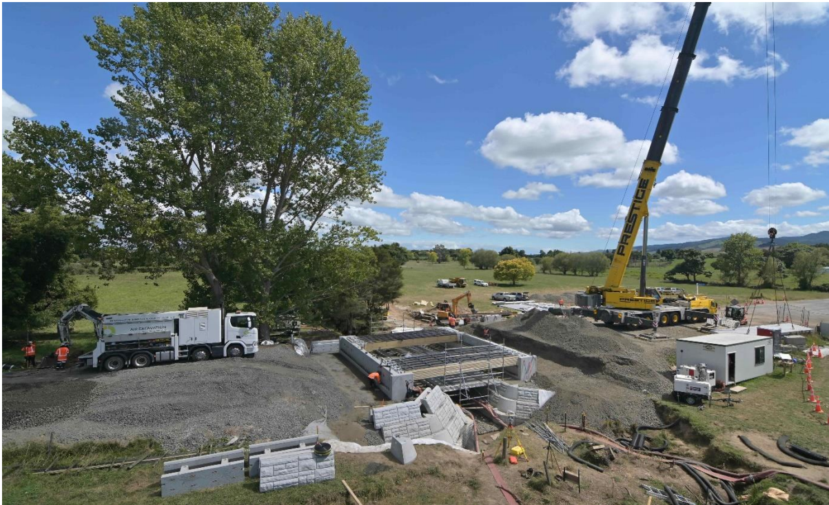
New Onetai Stream Bridge under construction
