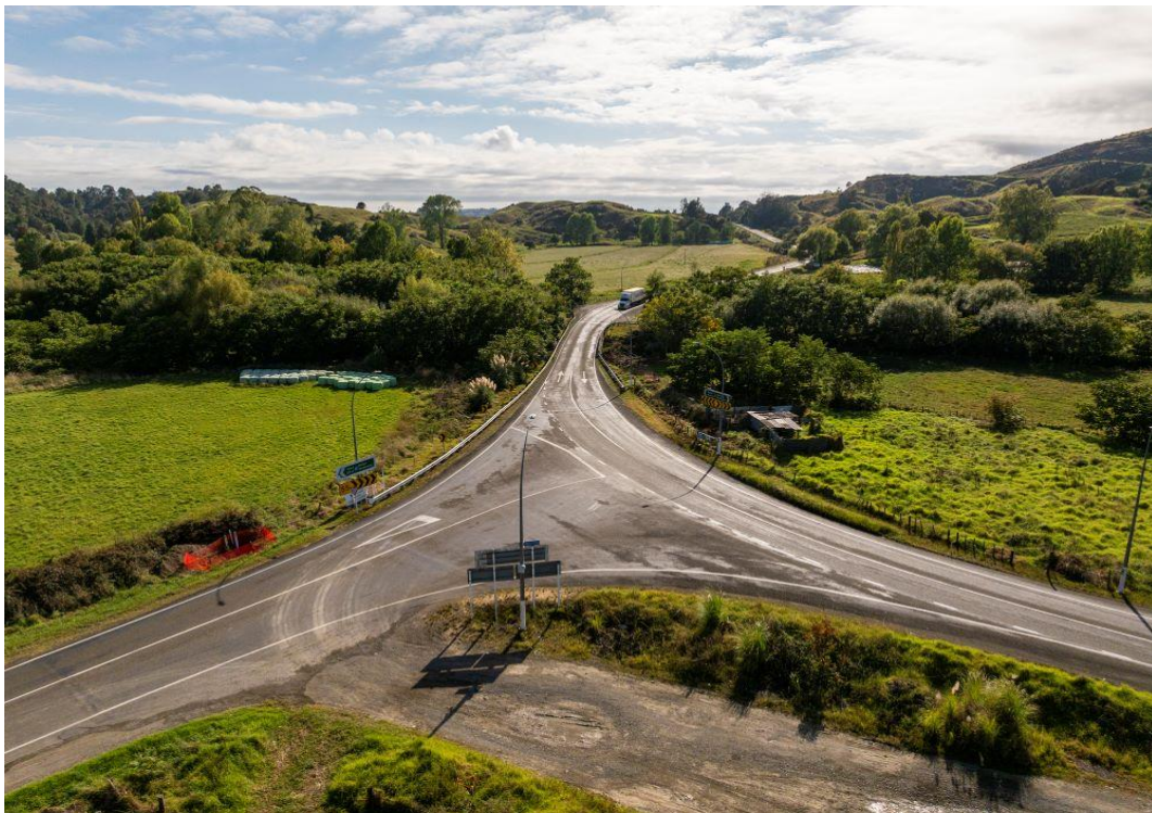
SH2/Wainui Road intersection
